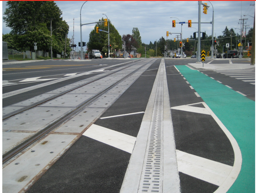
Monolithic polymer concrete 8" trench drain with high capacity intake slots and pipe connection flume.
