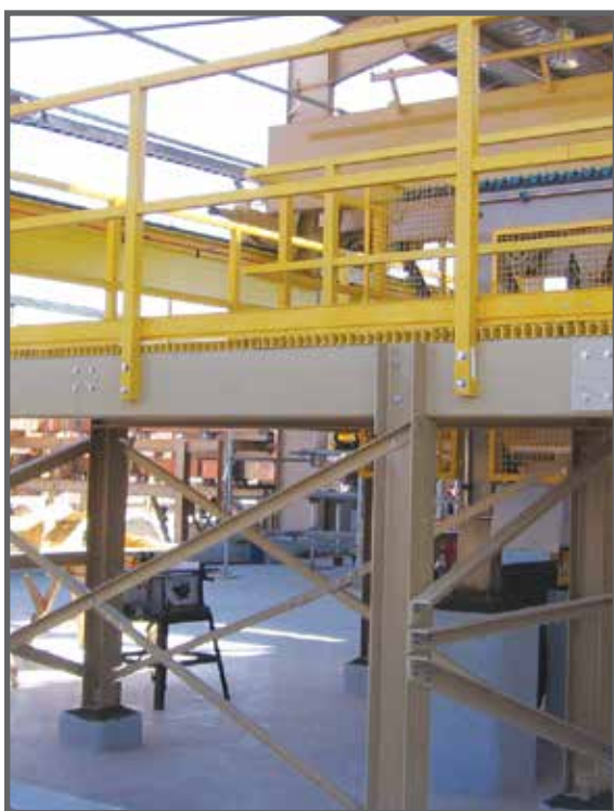
Fibergrate structural shapes and pultruded grating were used in this mining facility for their corrosion resistance.
