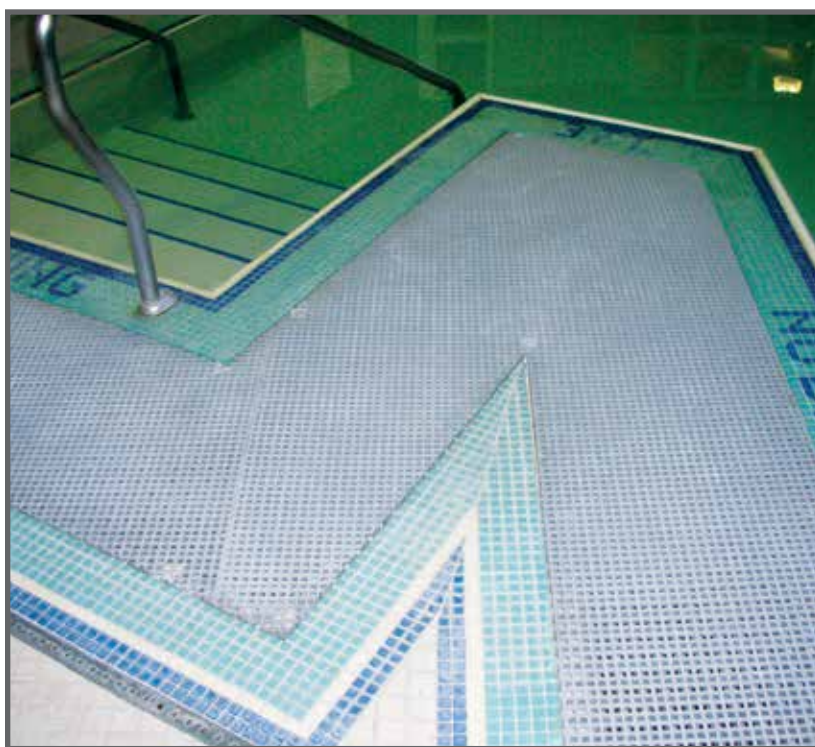
Fibergrate's Micro-Mesh® molded grating, found in this public pool, required detailed fabrication due to the curves and angles of the pool's design.
