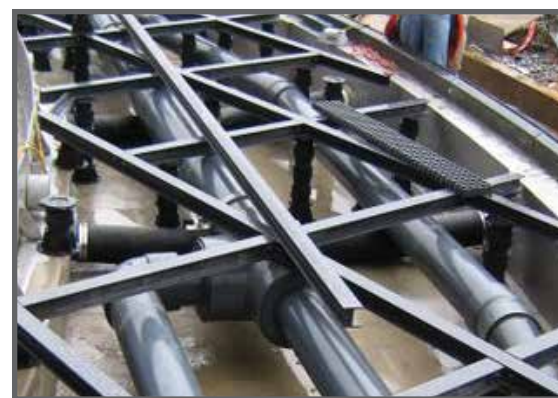
This fountain in Dallas required detailed fabrication of grating and structural components that could be submerged in water without corrosion or rust.
