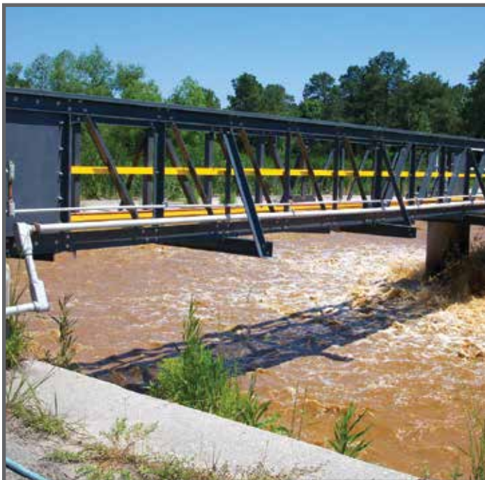
This all FRP truss walkway was designed and engineered to replace an existing rusted steel structure.
