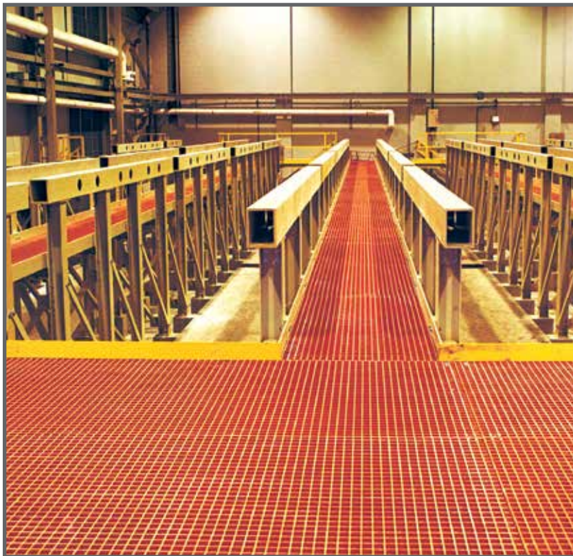
This battery plating facility's demanding corrosive environment required FRP elevated walkways, fabricated from Dynaform® vinyl ester structural shapes and Vi-Corr® molded grating.
