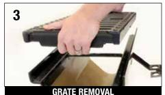
To remove grates use wrench or socket set. Carefully store bolts for refitting of grates.
